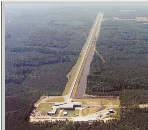
The Louisiana LIGO facility is located in a remote, flat location, relatively isolated from man-made noise. It has two massive, two-and-a-half mile long arms that form an "L" shape and contain steel pipes emptied of air. Laser light traveling through these arms is used to measure changes in the curvature of space.
